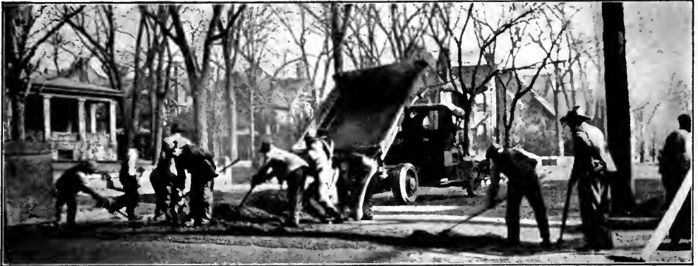
SPREADING SHEET ASPHALT FOR NEW SURFACE ON RESHAPED MACADAM ROAD
